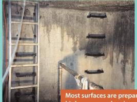
Most surfaces are prepared by high-pressure cleaning
